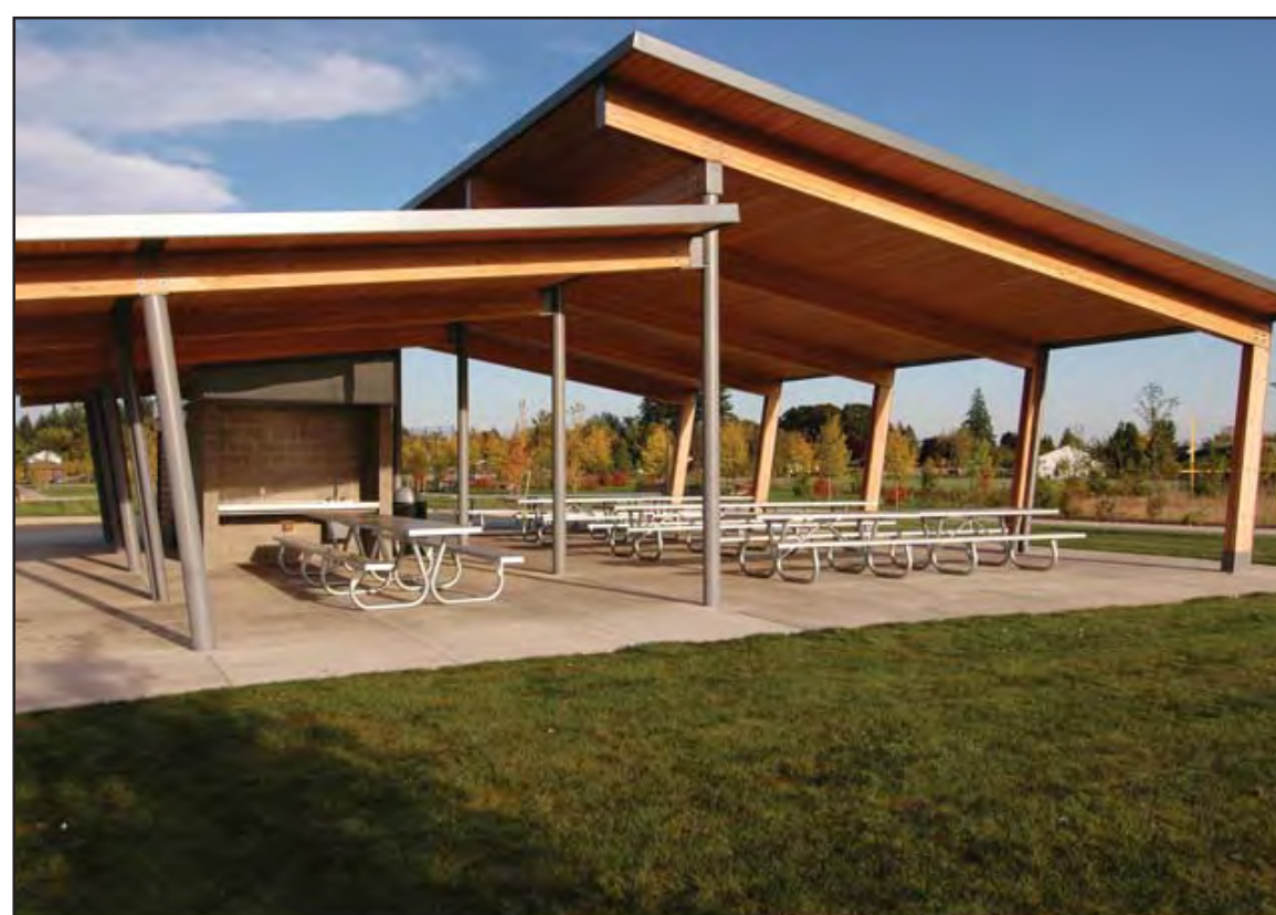
OPEN AIR SHELTER WITH RESTROOMS
